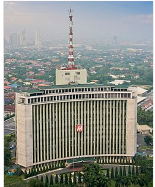
Meralco (López) Building along Ortigas Avenue, Pasig, Metro Manila .
